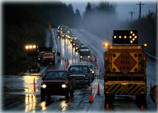
Work Zone Location/Status
